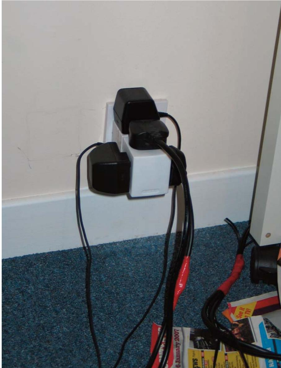
Plate 4 Demonstration of High Risk Wiring
